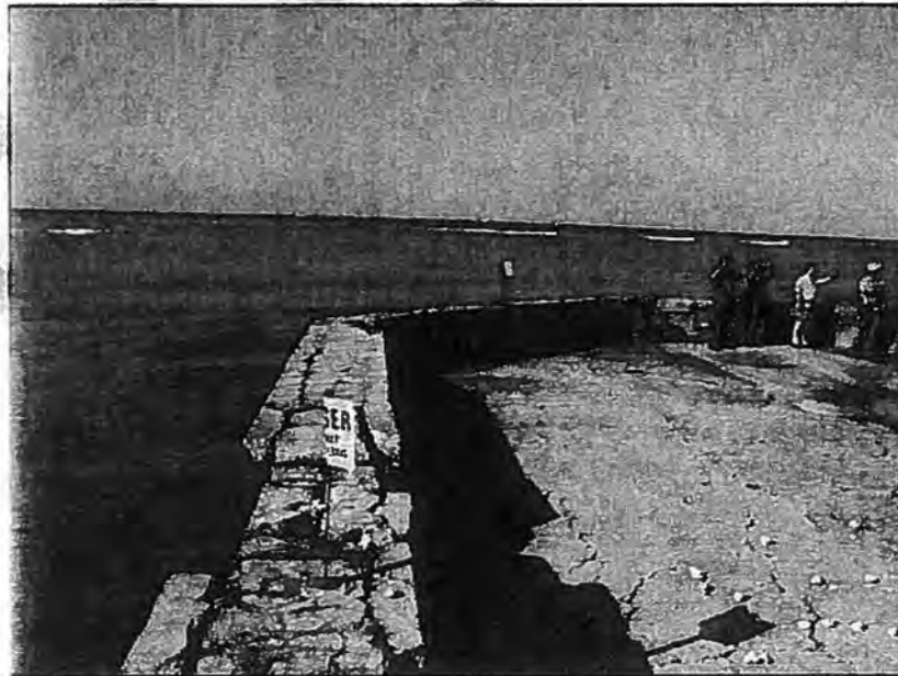
Plate 7. Cracked and Crumbling Perimeter Seawall, 2007
