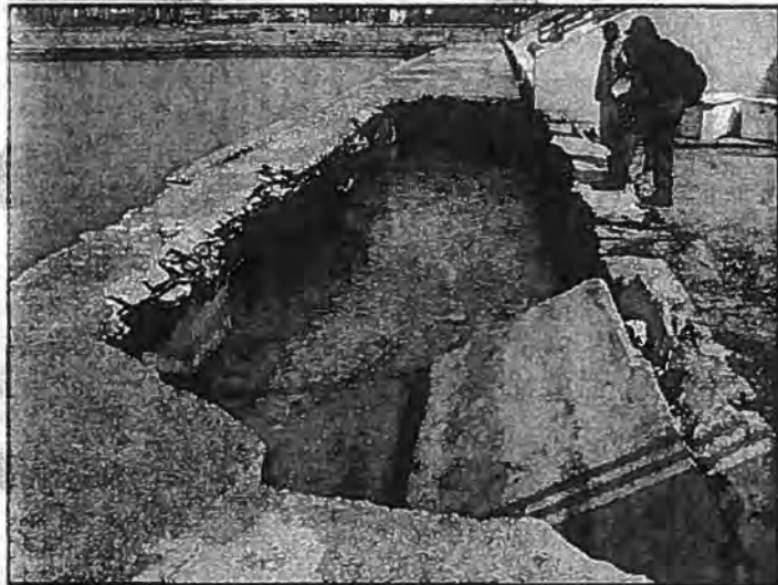
Plate 9. Collapsed Mauka Deck in Front of the Triple Arch Entry, 2006
