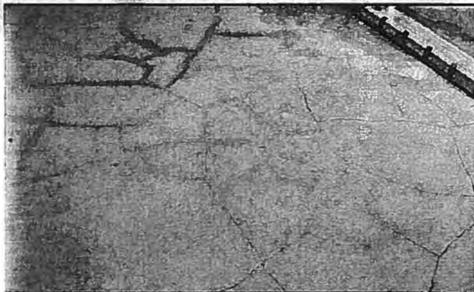
Plate 14. Cracks in the Restored Slab-on-Grade Concrete Floor, 2006
