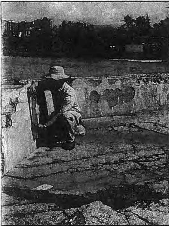
Plate 5. Seawall Tilt, 2007 The tilt from vertical indicates that the top of the seawall is rotating seaward.
