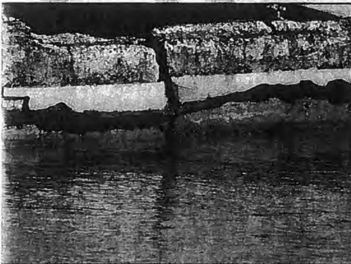
Plate 10. Cracked Ewa Deck, 2007
