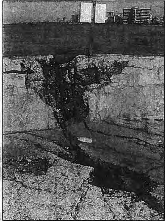
Plate 6: Cracked Seawall Ewa corner and Deck, 2007 The crack extends the entire width of the seawall and continues across the deck to its inner edge.
