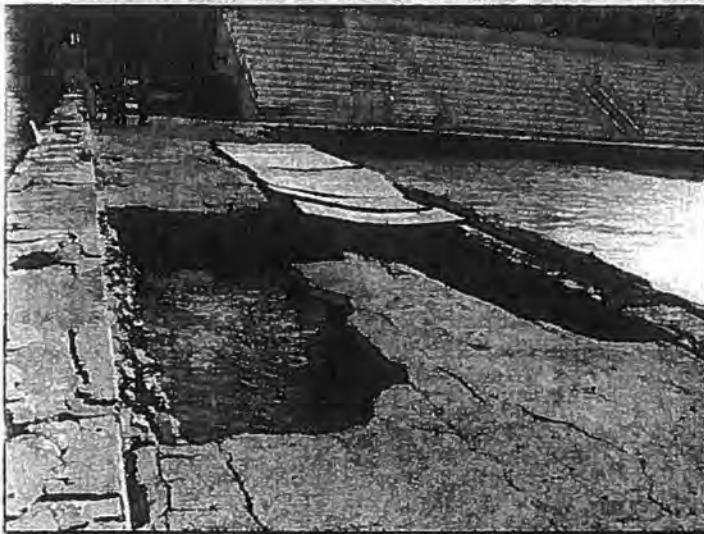
Plate 8. Collapsed Ewa Deck, 2007
